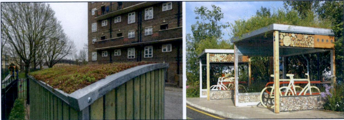
Figure 3: Examples of (left) green roof bin store systems and (right) green roof and integrated insect hotel bike stores
