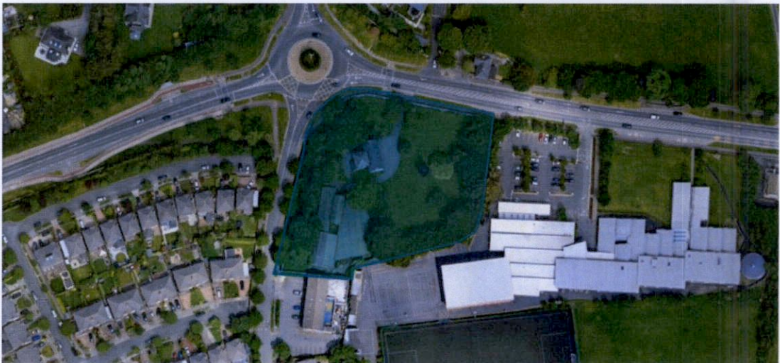
Figure 1.1 – Aerial View of Site and Surrounding Context
