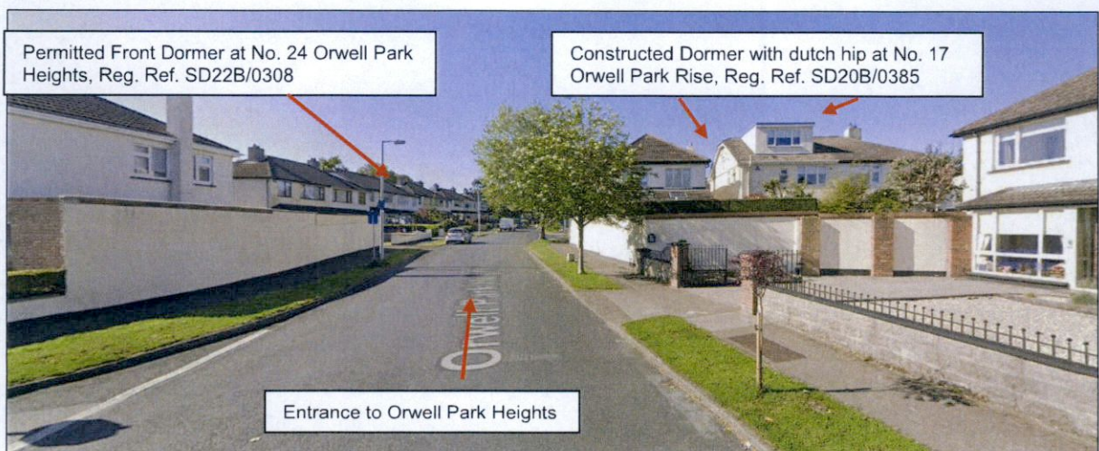
Figure 5.0 Street view of 2 no. dormers visible entering Orwell Park Heights.
