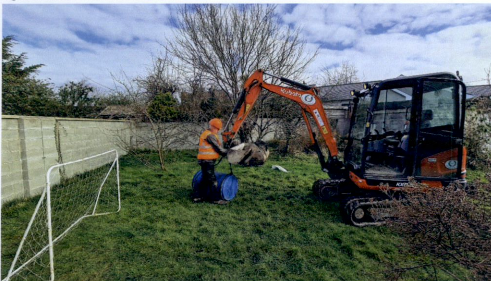
Fig 3. Site View North
