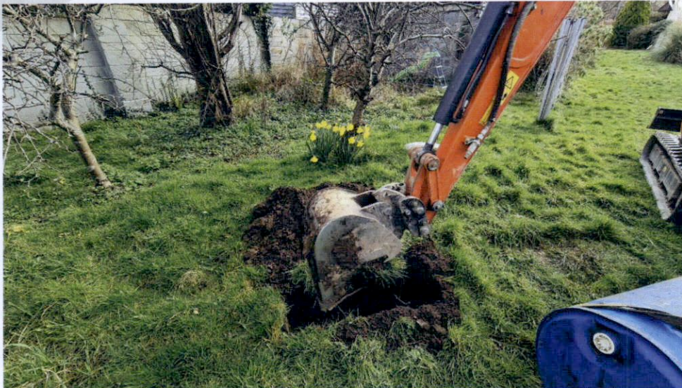
Fig 7. Infiltration test location 22-02-2023
