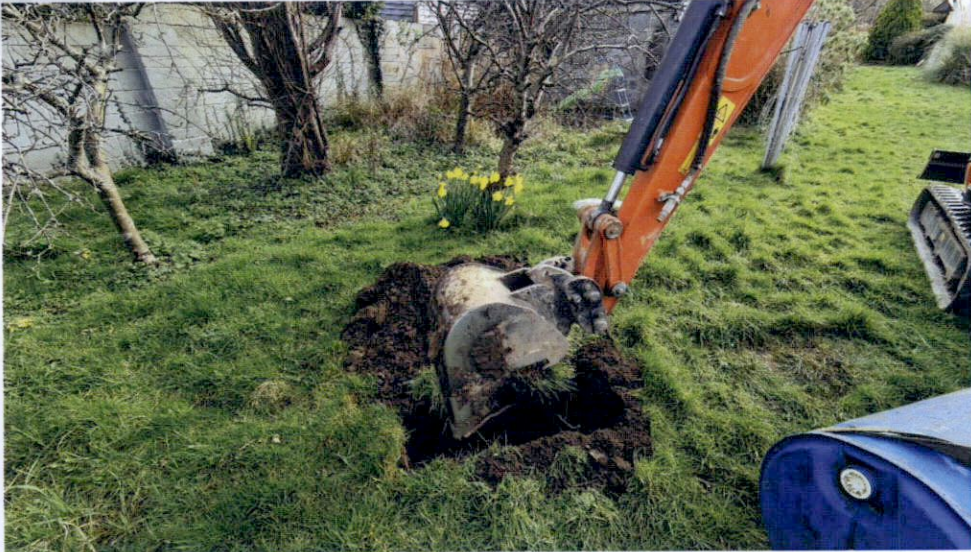
Fig 7. Infiltration test location 22-02-2023
