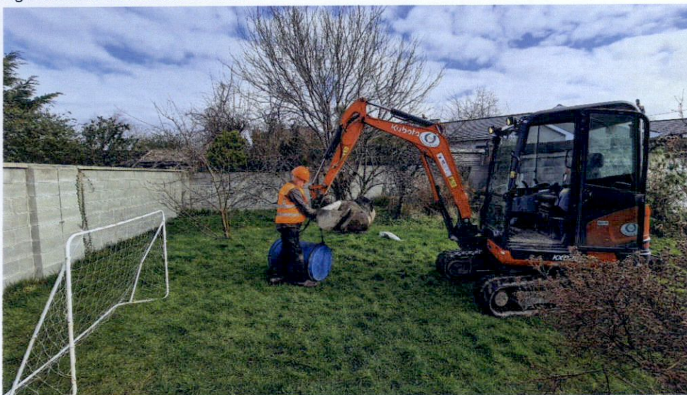
Fig 3. Site View North
