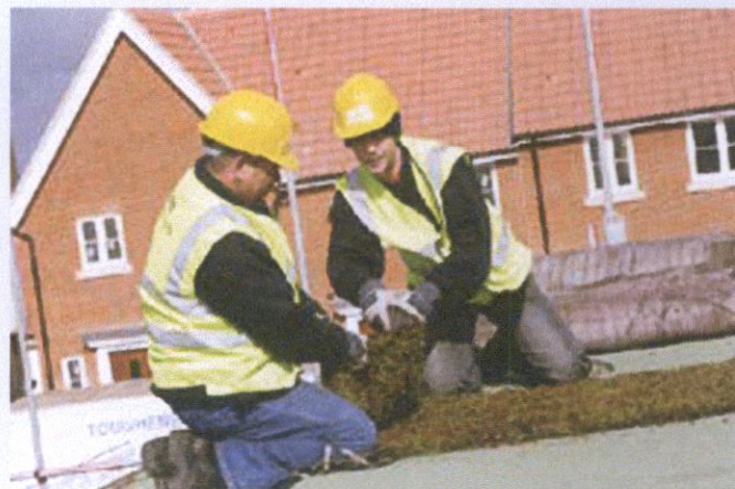
Short 2m rolls of XF301 Sedum System installed by hand.
