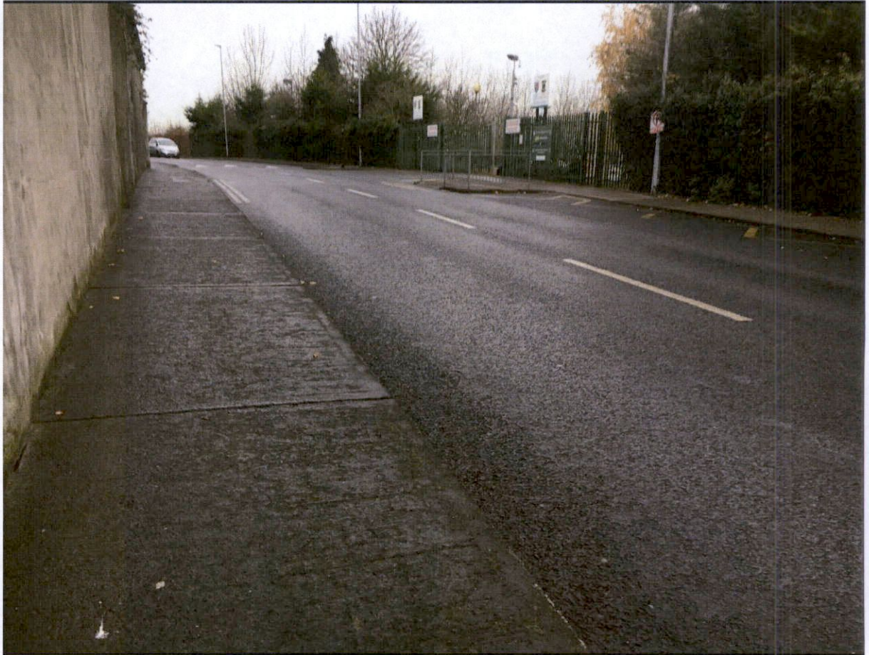
Photograph 5 – Existing gated school access
