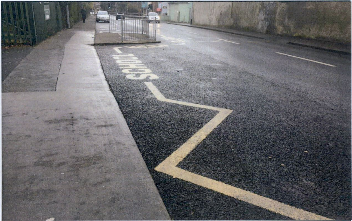
Photograph 3 – Existing road markings at the school access
