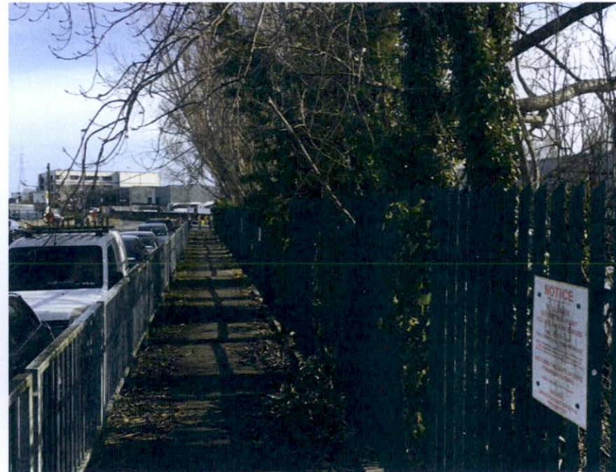
Northern flat bar railing boundary - facing east
