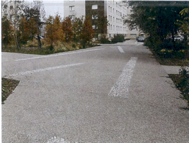
Residential courtyard with exposed aggr concrete surface and tree planting
