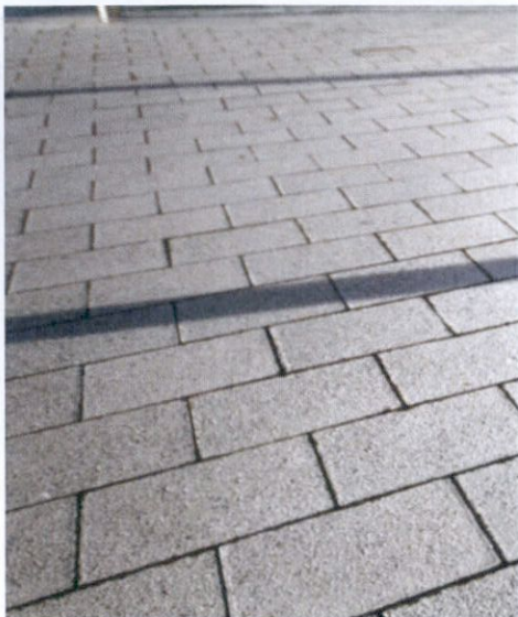
Core building entrance paving - Silver granite PCC pavours
