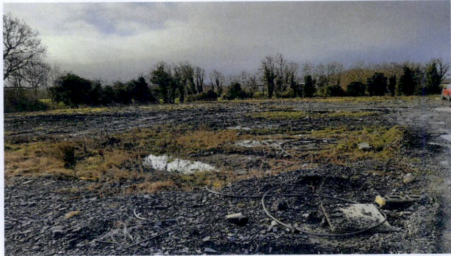
Picture 5: View of existing site – direction of view: West.
