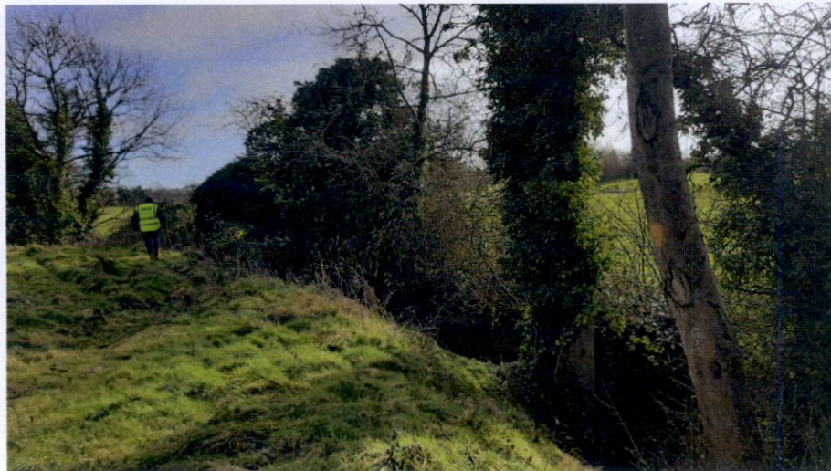
Picture 11: Picture of the existing ditch along the South site boundary
