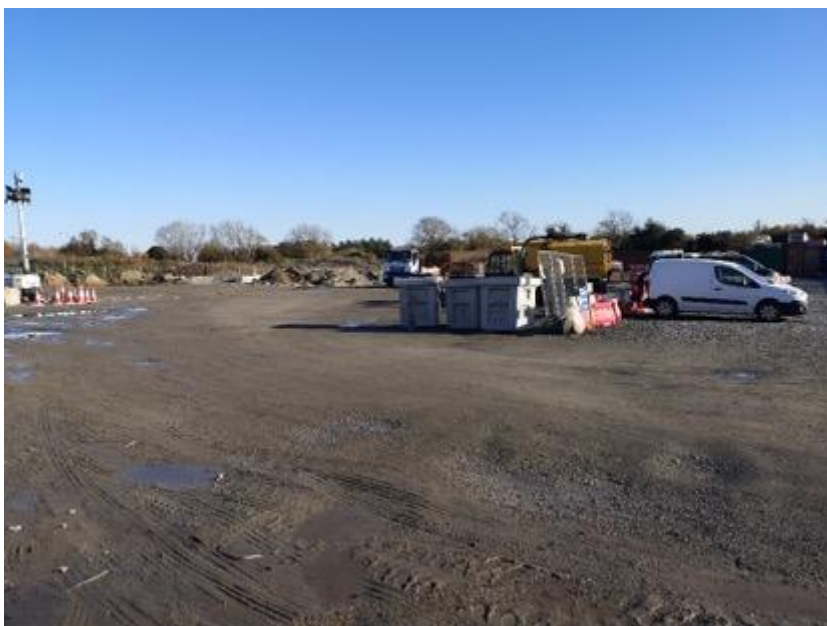
Figure 15.14. View of hardcore area from southwest
