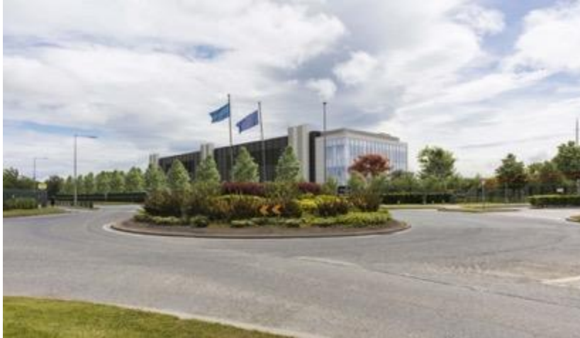
Figure 3.6 - CGI of Proposed Data Centre from New Nangor Road R134 in Profile Park
