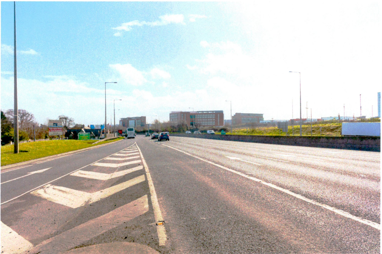
Fig. 11; Extract of CGI image, with view from N4 looking east, prepared by Digital Dimensions.
