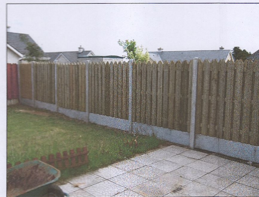
2000mm high vertical timber fencing panels with concrete plinth and post
