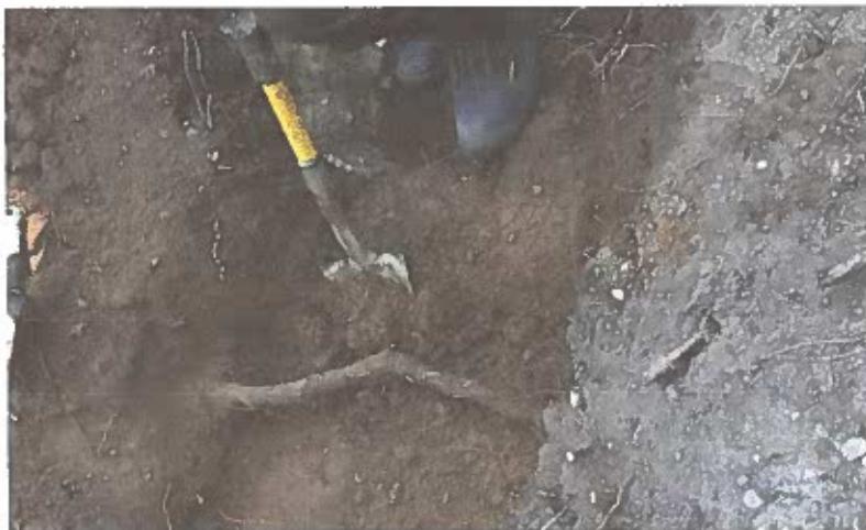
Photo 1: Hand excavation around the root to be retained within the pit.
