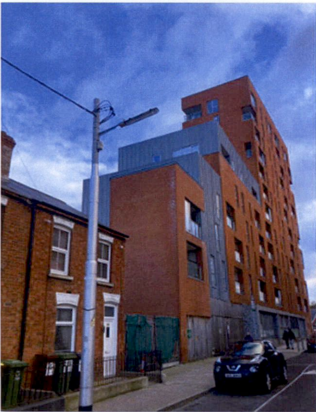
Drimnagh Road, Dublin 12
