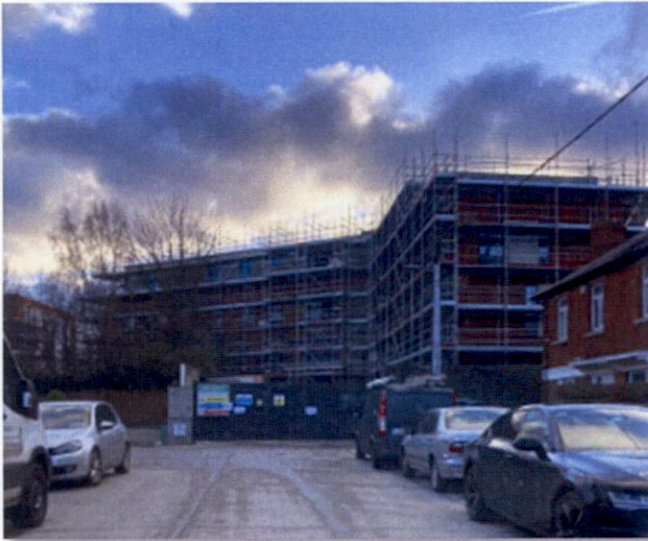
Parnell Avenue, Dublin 12 Canal
