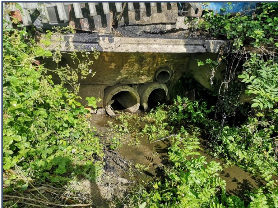
**Figure 5-8 Inlet to twin-pipe culvert**
