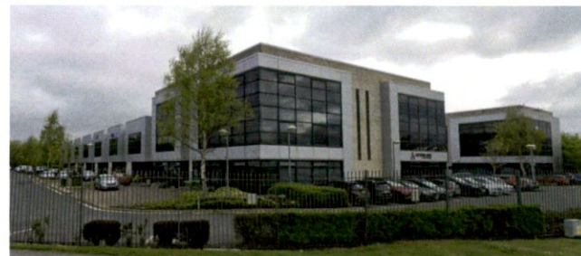
Figure 5 – Photograph of Neighbouring Building in the Immediate Vicinity of the Proposed Development
