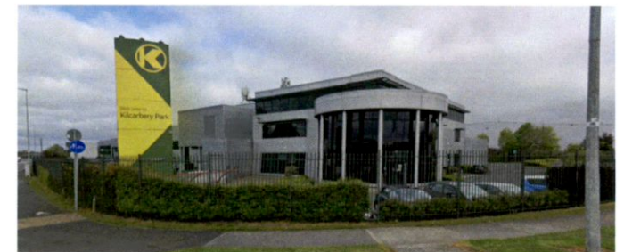
Figure 6 – Photograph of Neighbouring Building in the Immediate Vicinity of the Proposed Development
