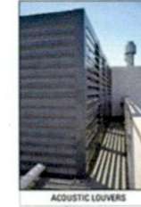
Figure 33 – Screening To Plan on Roof
