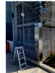
Figure 29 – Mesh & Green Wall To External Stair Core
