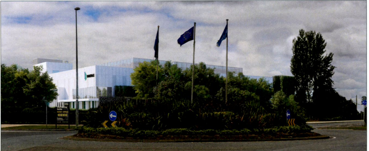
Photomontage of revised elevations of proposed development as submitted under this AI submission in year 5 after completion
