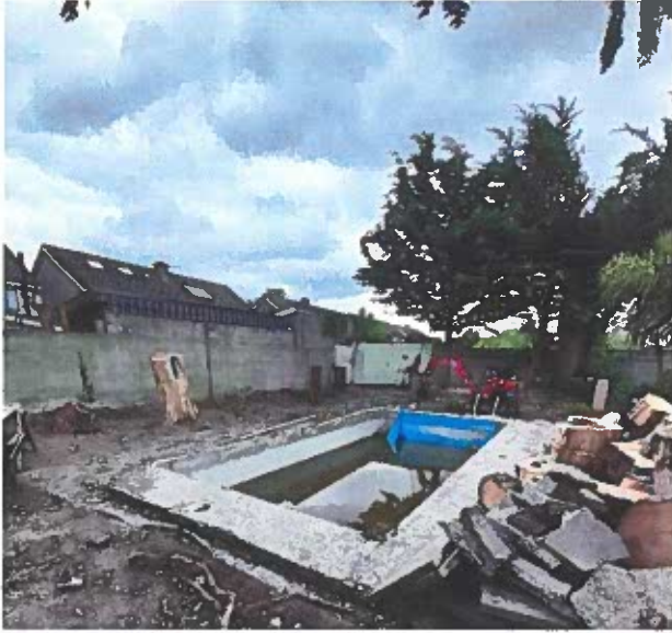
Photo A1 (Looking to the East)
