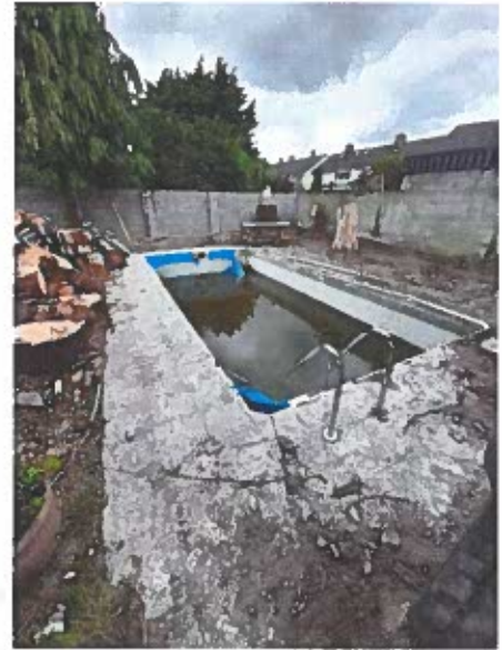
Photo A2 (Looking to the West)
