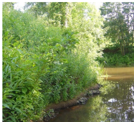
Fig 5 - Living willow wall 3 years after installation
