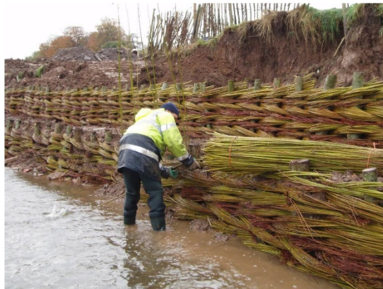
Fig 4 – Living willow wall installation
