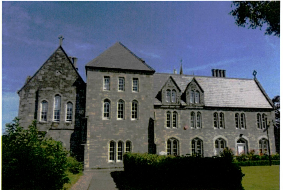
Fig 6: Elevation / view of the south-facing wing : the more utilitarian nature of the three-storey wing is expressed externally with simpler windows and a greater proportion of masonry. The raised wall dormers with paired windows break up the mass of an otherwise large area of plain slate roof.
