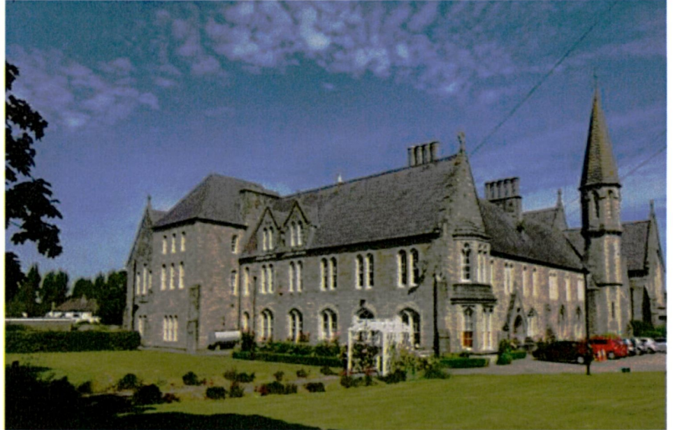
Fig 5: General view from south-east showing the east facing wing and its conjunction with the south facing wing (composed of two and three storey elements).
