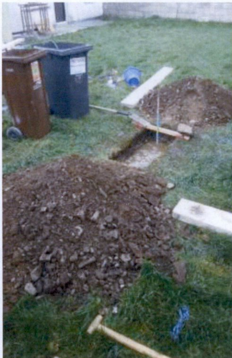
Arisings from Test Pit
