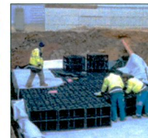
Industrial building, Tumelstham (AT)
