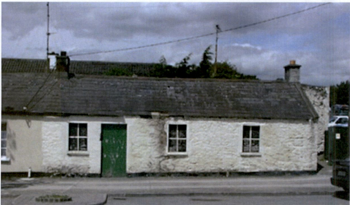
Figure 4: Front Façade to Rathcoole Main Street
