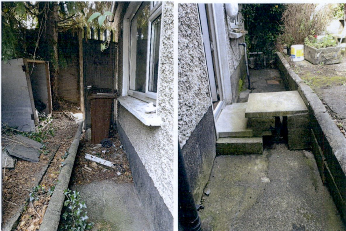
Figure 9: North (Rear) Elevation
