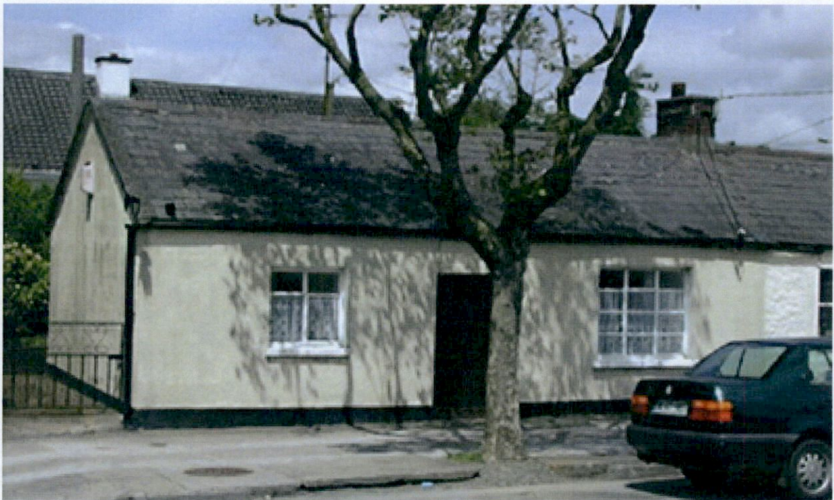
Figure 5: Front Façade to Rathcoole Main Street
