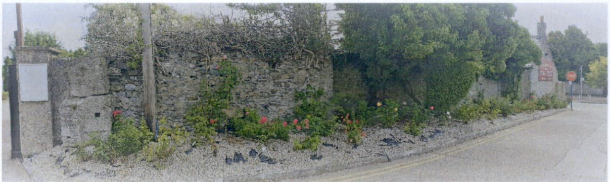
Figure 13: Western Boundary Wall
