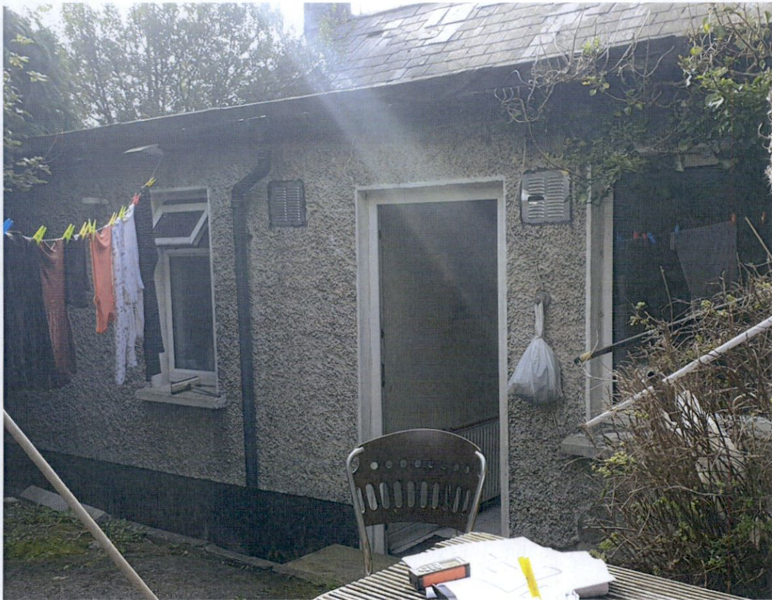
Figure 8: North (Rear) Elevation
