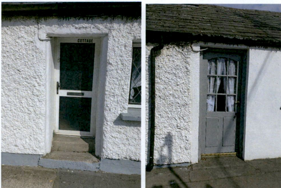
Figure 7: South (Front) Elevation Entrance Doors Detail
