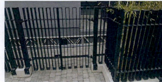
1.8m high steel railing fence with access gate - To enclose private courtyard space.
