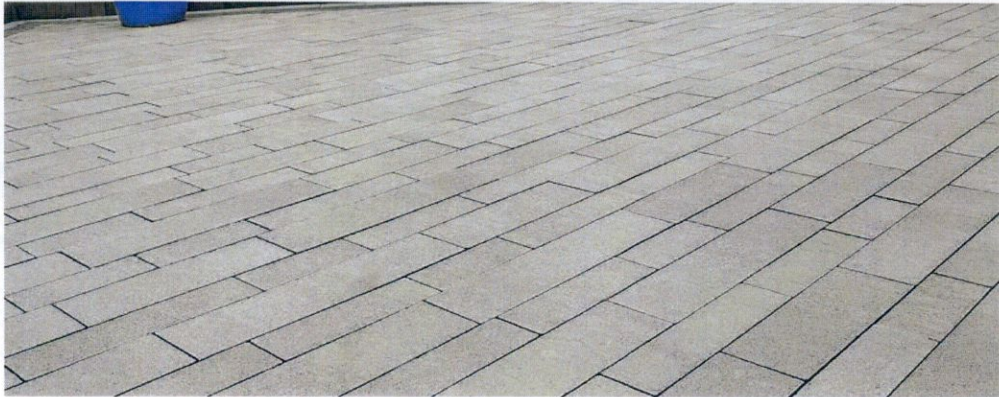
P1 - PROPOSED CONCRETE BLOCK FLAG PAVING - COLOUR: NATURAL GREY, SIZE: 600 X 200 X 50mm, OR SIMILAR APPROVED, STAGGERED BOND PRODUCT: PEMBROKE FLAG BY ROADSTONE OR SIMILAR APPROVED.
