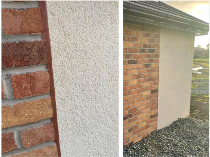
Primula brick with grey mortar and buttermilk render (Vandersanden or similar approved)
