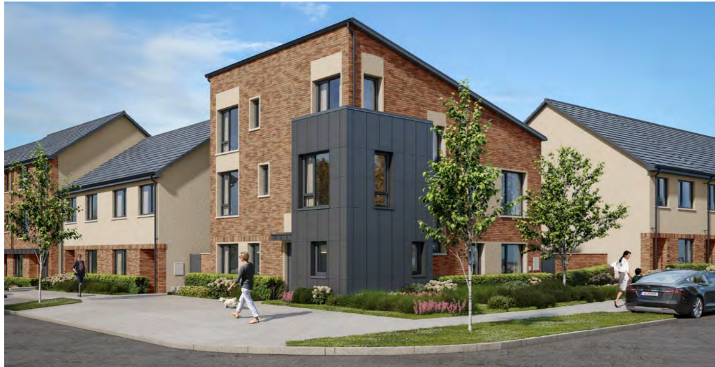
Revised Landmark Building B - View (A) looking north
