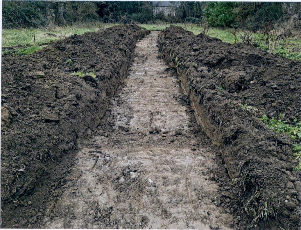
Plate 13 Trench 8 Looking South
