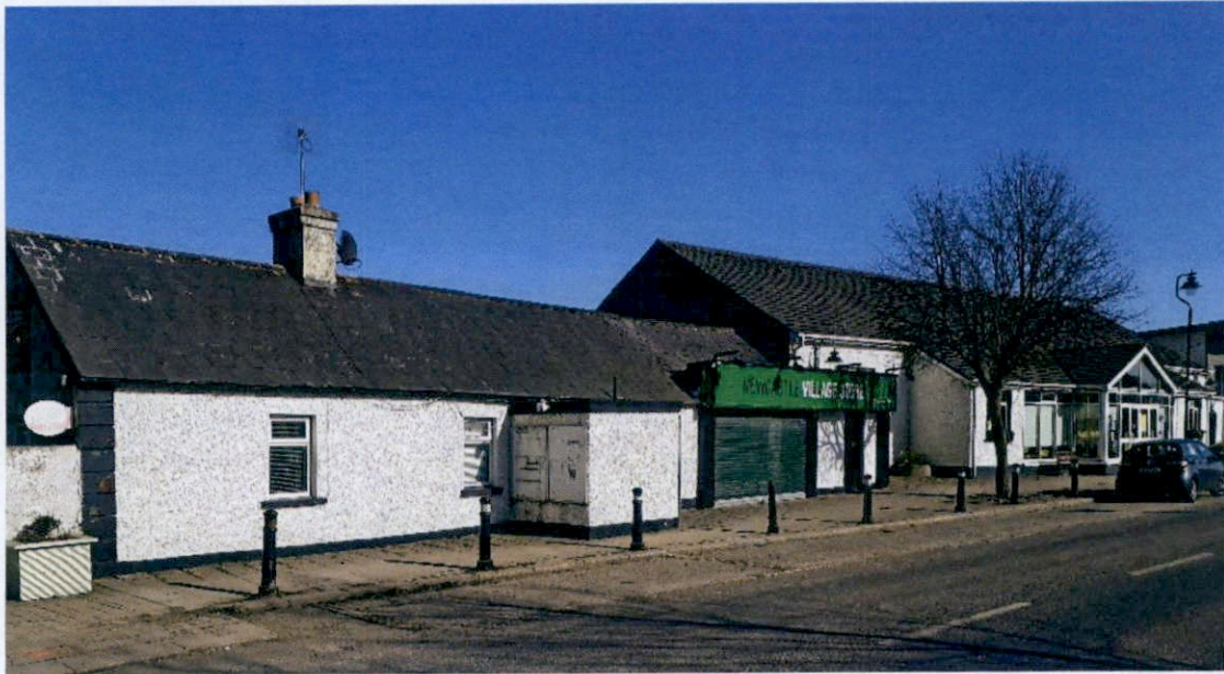
Plate 1 Existing Buildings at Front of Site
