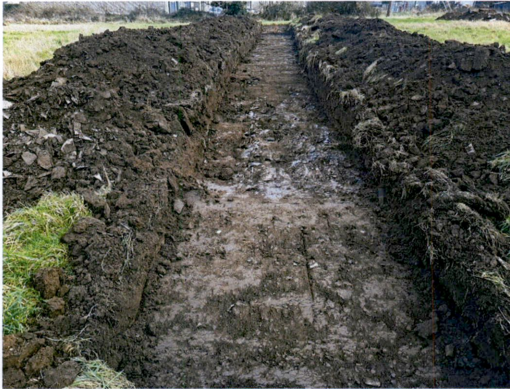
Plate 7 Trench 2 Looking East
