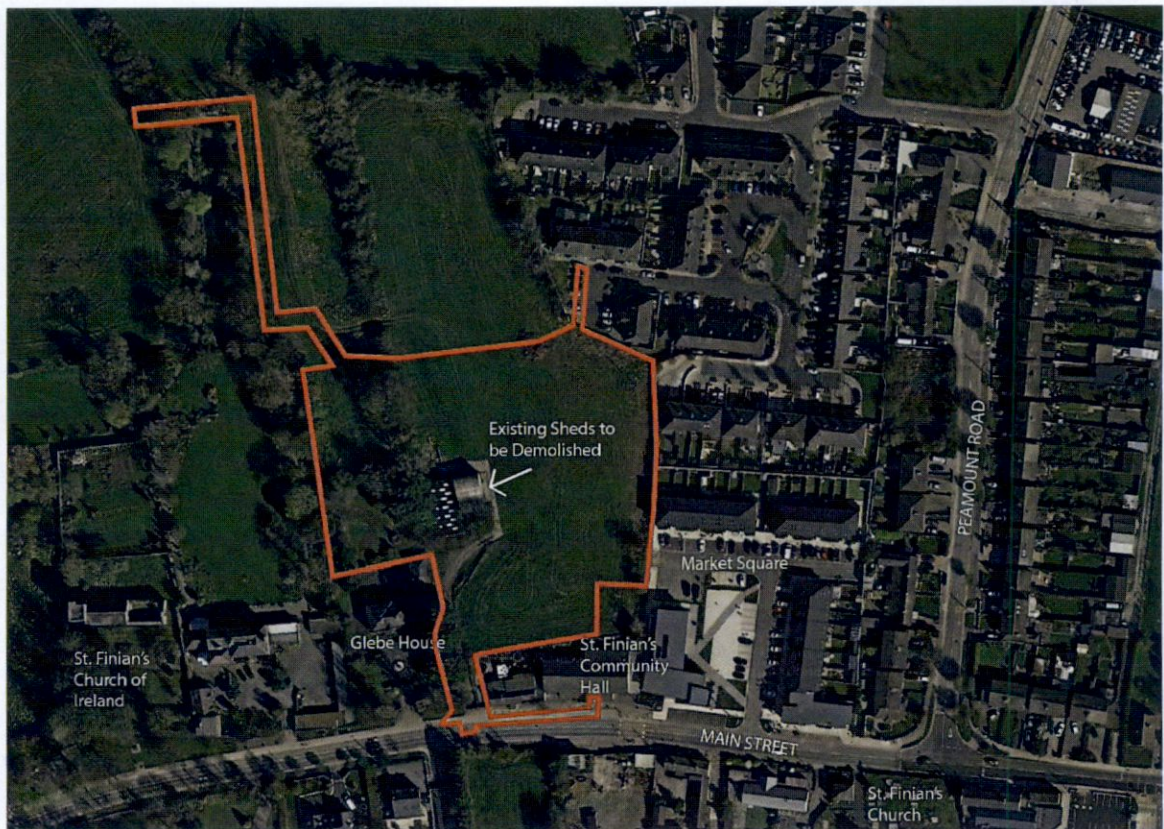
Aerial View of Existing Site
