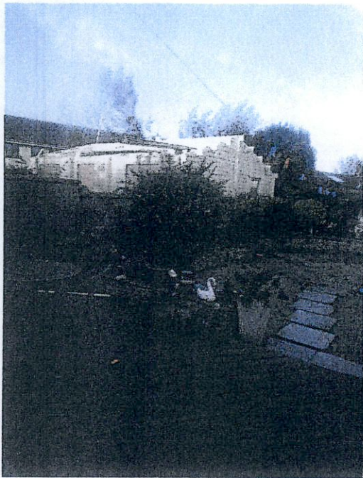
Photo No 3 View from No 7 Aranleigh Gardens During Construction
