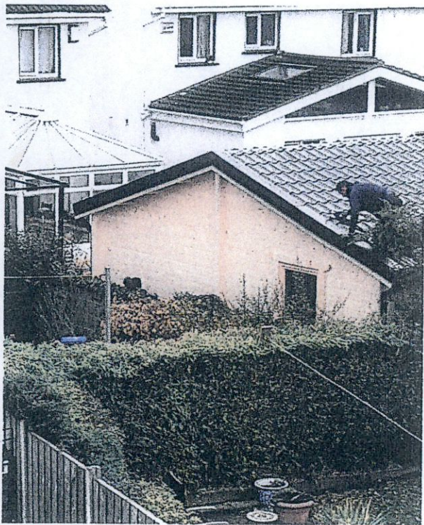
Photo 8 View from 2 Aranleigh Court – under Construction
