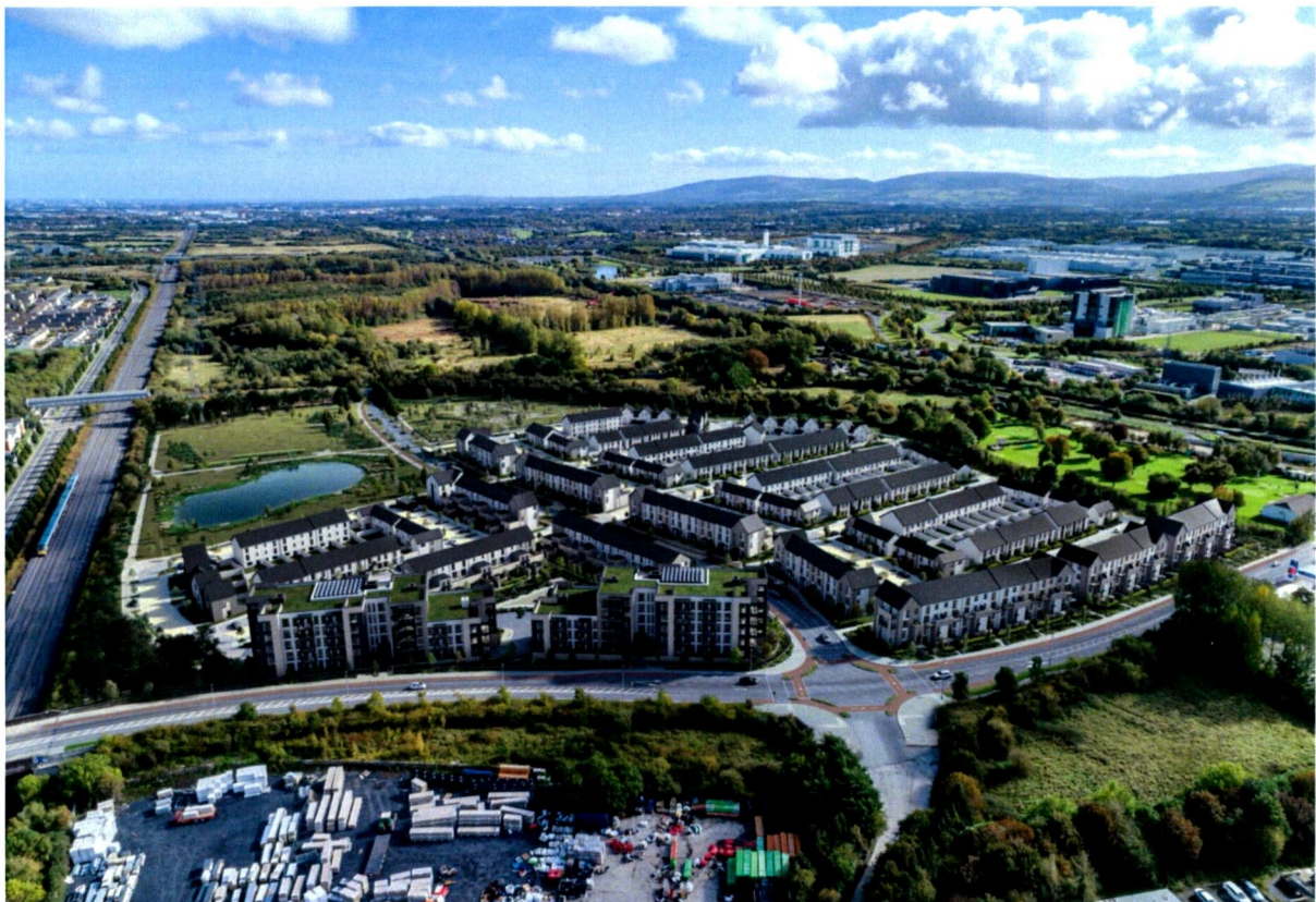
Figure 4: Computer Generated Image, prepared by 3D Design Bureau showing an aerial view the proposed development with the permitted road and infrastructure works show.
