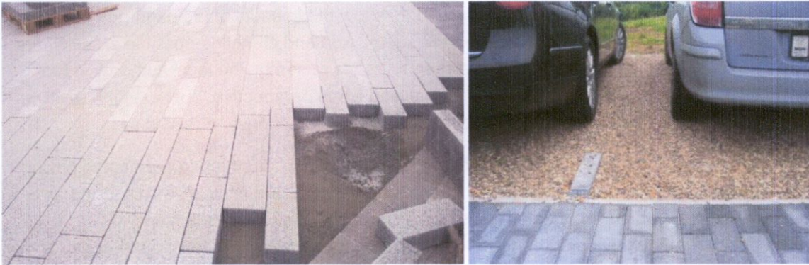
Figure 1. Pre-cast concrete unit paving, laid with proprietary spacers. Figure 2. 'Nidagravel' grid filled with angular gravel
