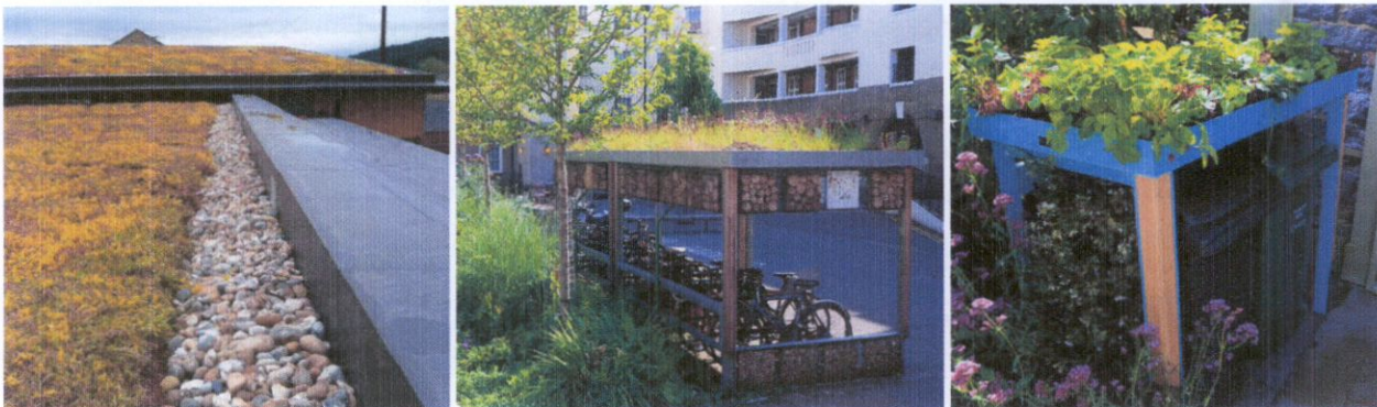
Figures 4-6. View of typical extensive 'sedum' roof; view of green-roofed cycle shelter by GreenRoofSheltersUK; and view of green-roofed bin shelter by FrontYardCompanyUK
