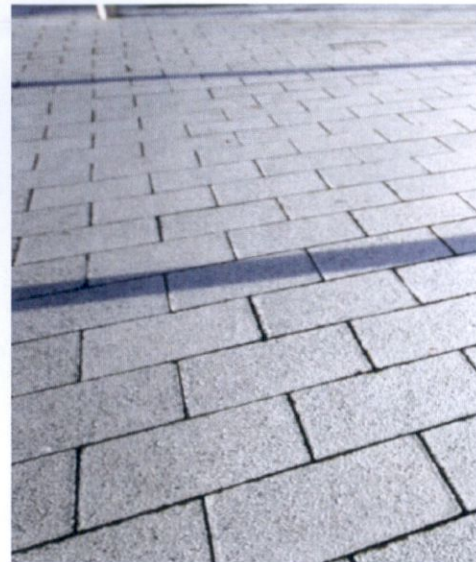
Core building entrance paving - Silver granite PCC pavours
