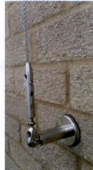
Jaw tensioner attached to pro-eye fitting
