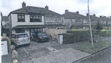
Description: Front side garden fence for height above 1.2m.
