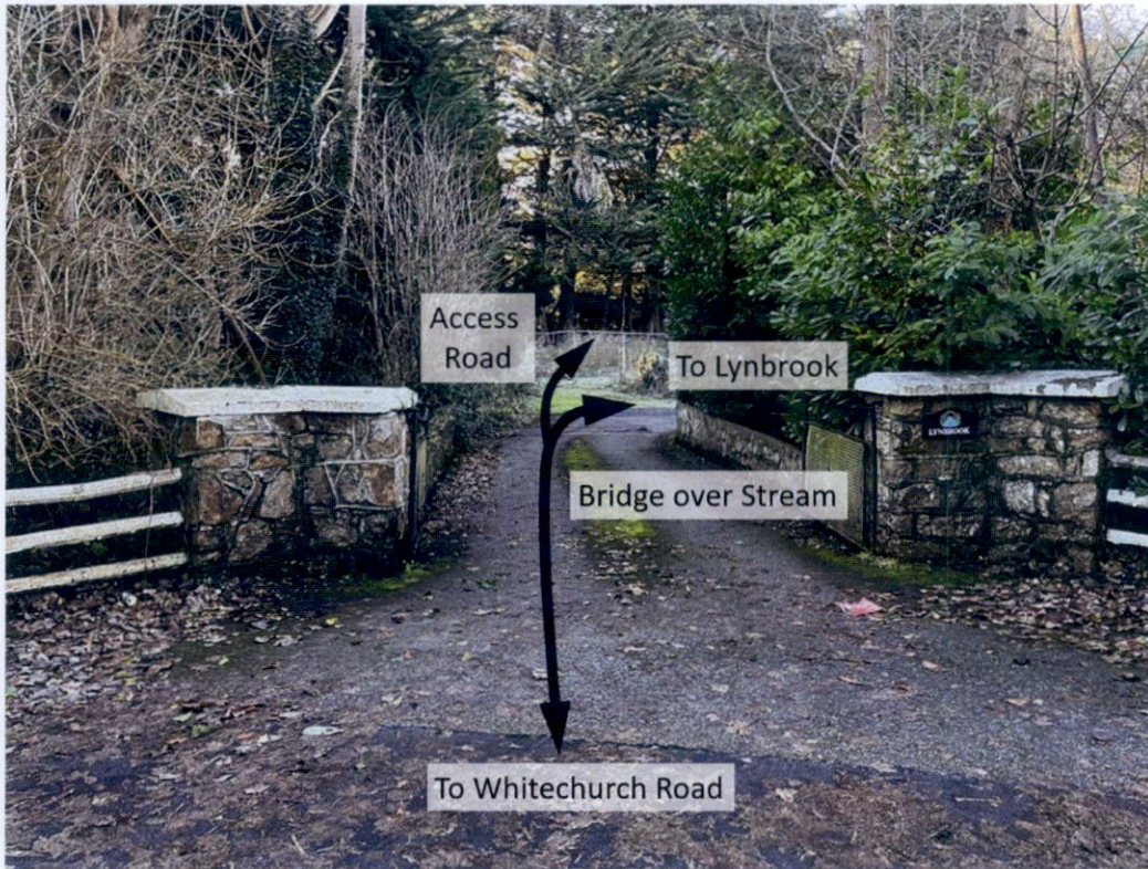
Image 02_Looking West towards "bridge" & access road from Whitechurch Road
