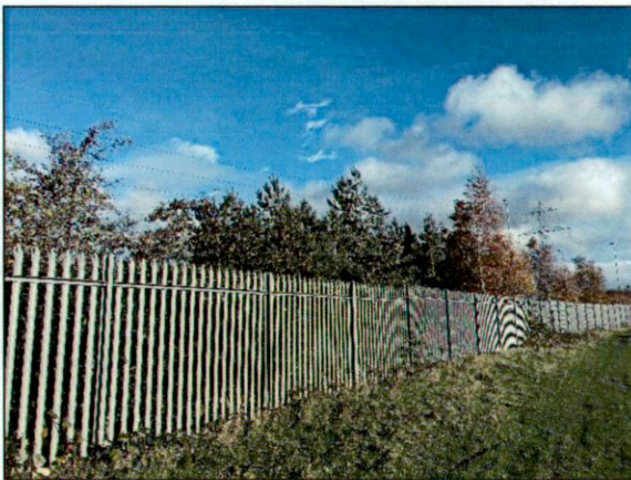
Plate 3 Tall palisade fencing to the north.
