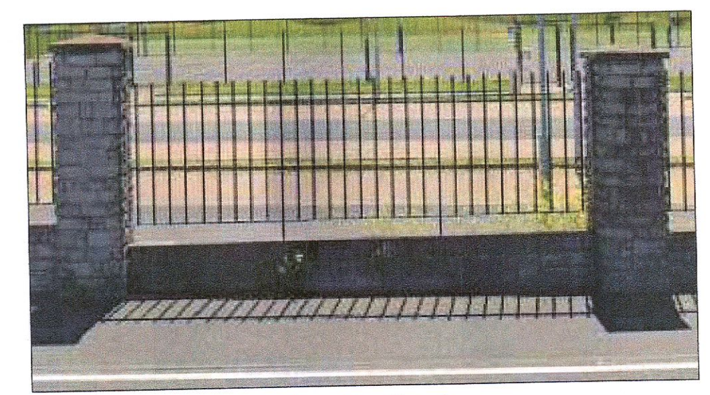
Sample image of existing wall & railing - Type A
