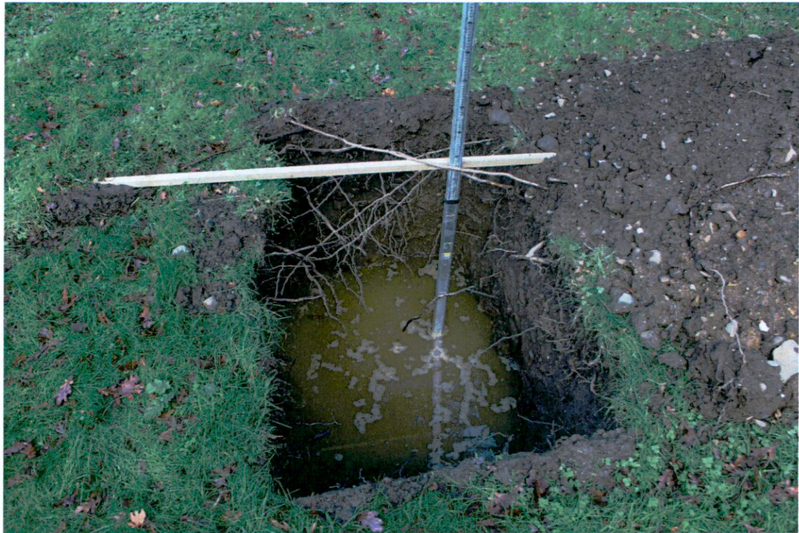
PHOTOGRAPH NO. 1 - TRIAL PIT NO. 1
