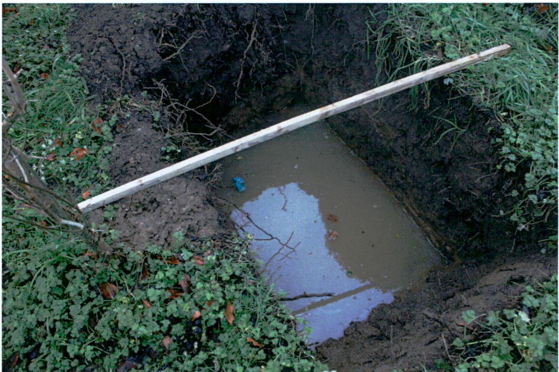
PHOTOGRAPH NO. 2 - TRIAL PIT NO. 2
