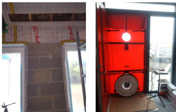
Figure 3: Air Tightness Testing Examples
