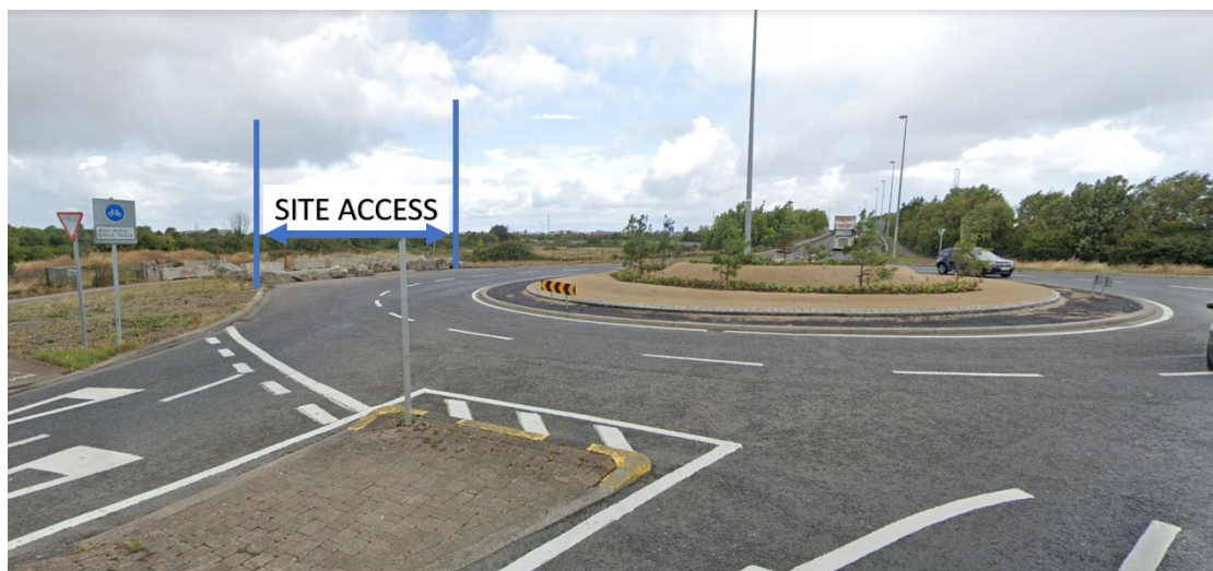
Figure 2-2: Access location from R113
