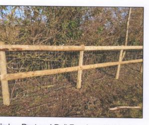
Timber Post and Rail Fencing with Mesh
