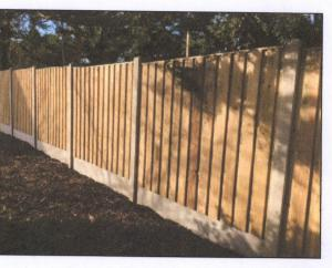
Concrete Post and Timber Panel Fencing
