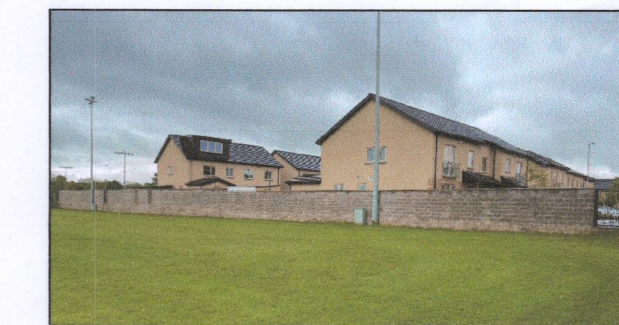
Existing Block Wall on Southern Boundary
