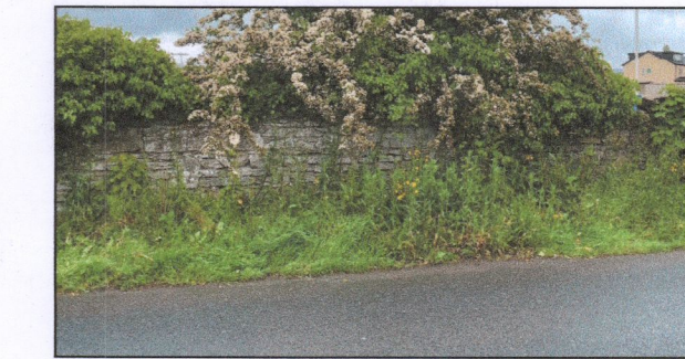
Existing Stone Wall Along Roadside
