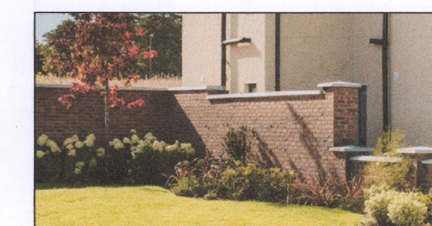
Concrete Block Wall with Brick Cladding
