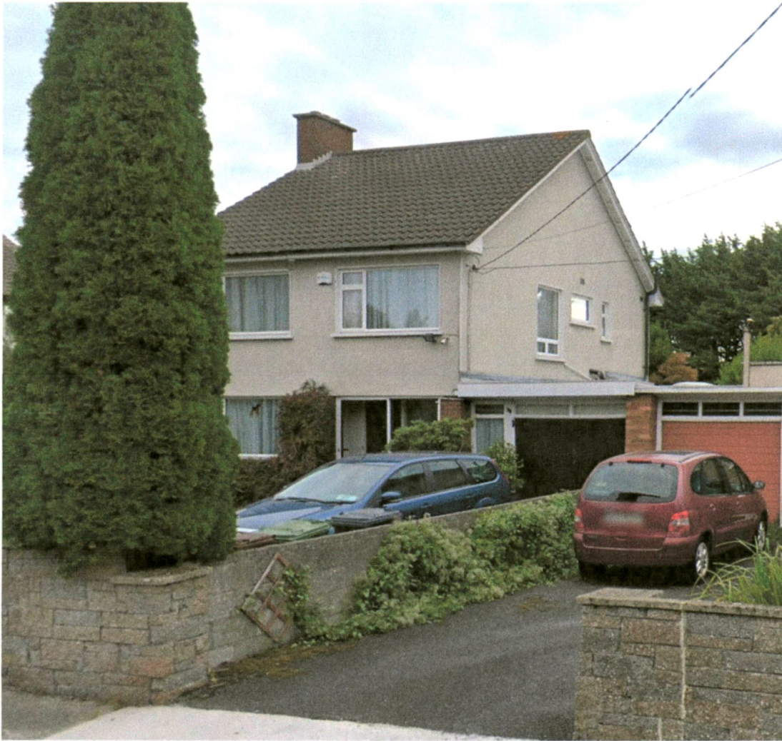
76 Crannagh Road- Gable ended
