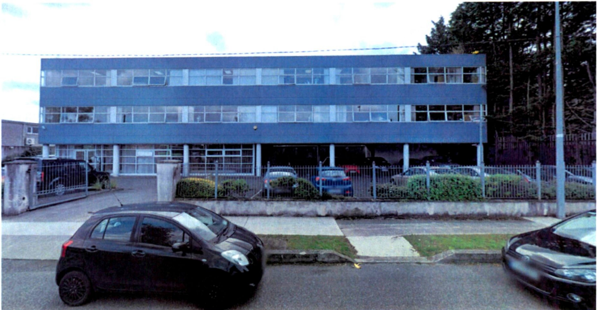
Figure 2: View of the existing building on site from Knockmitten Lane
