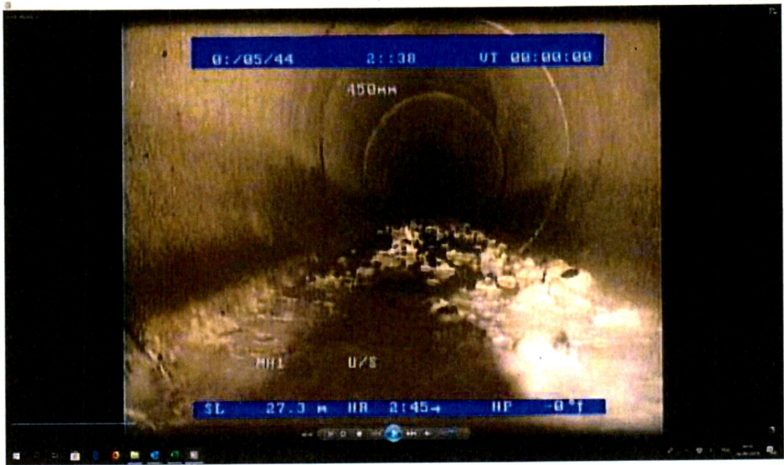
Debris & standing water. No connections
