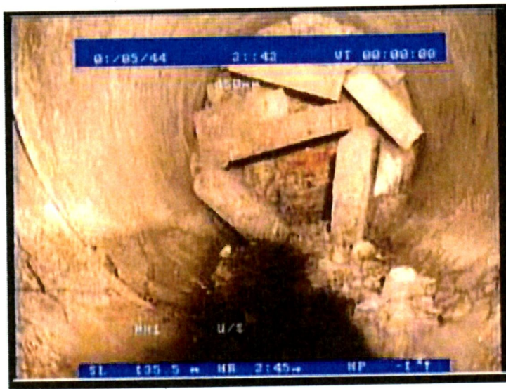
Fig. 7 - Snapshot from Camera Survey at termination.
