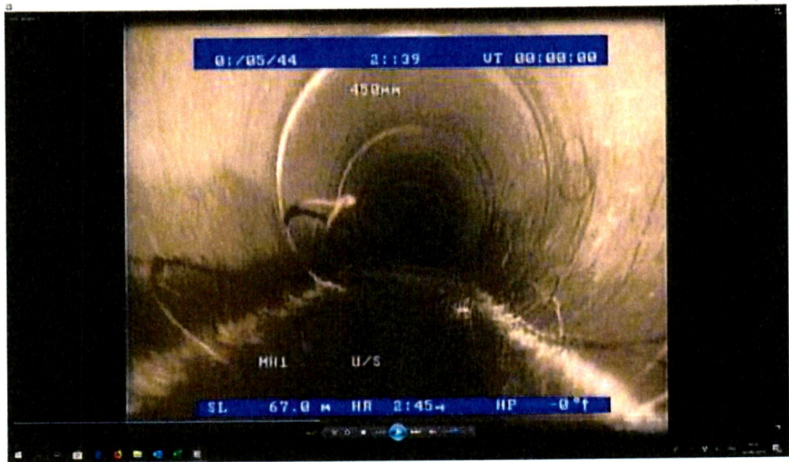
Extensive root growth. No Connections
