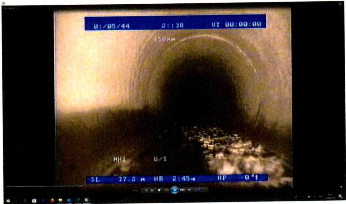
Debris in pipe. No connections
