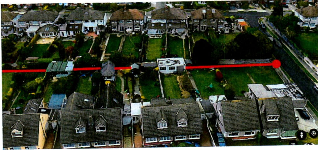
Fig 6 - Extract from google maps 3D view with the culvert line plotted, running under existing buildings
