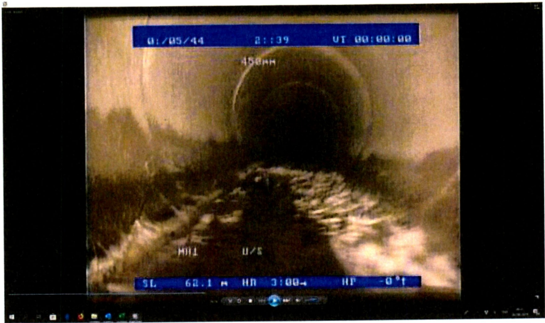
Extensive root growth. No Connections
