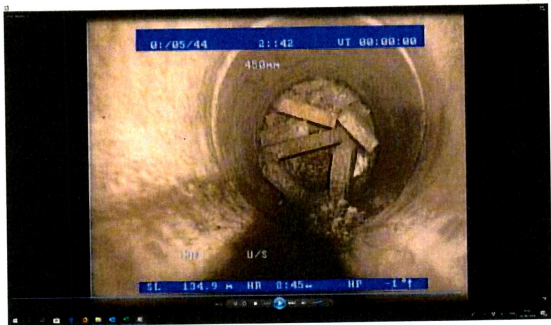
135m Termination of pipe. Blocked up with brick, block and concrete.
