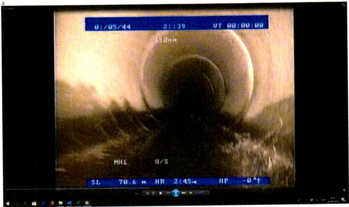
Extensive root growth. No Connections
