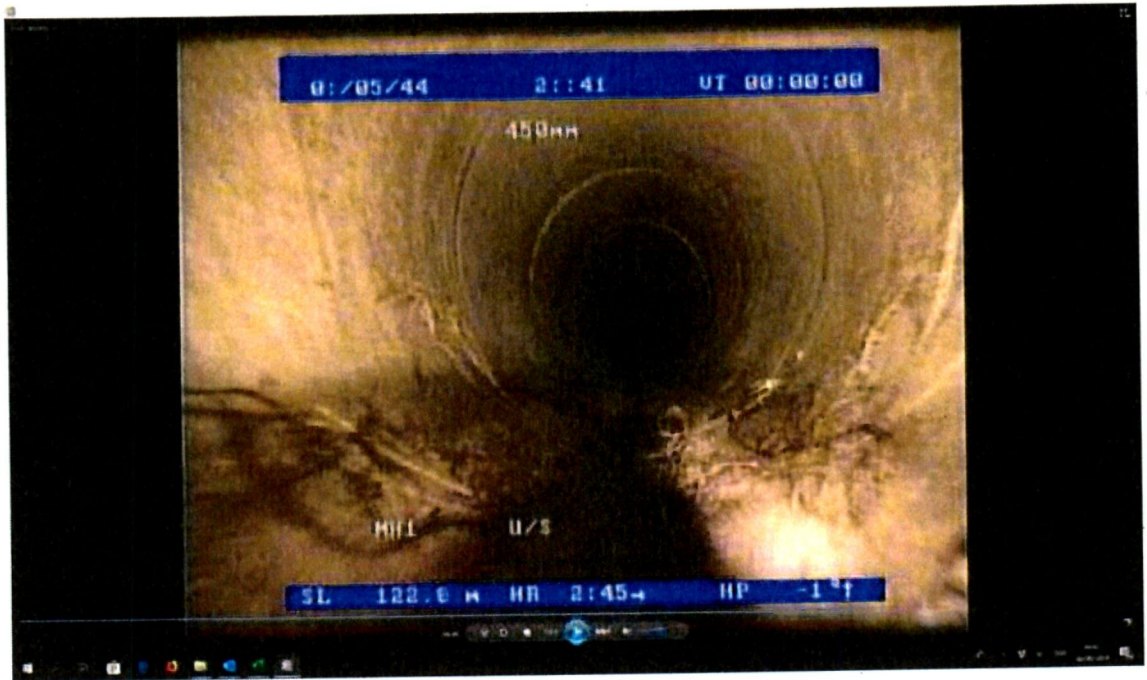
Distance 122.8m. Root growth. No Connections
