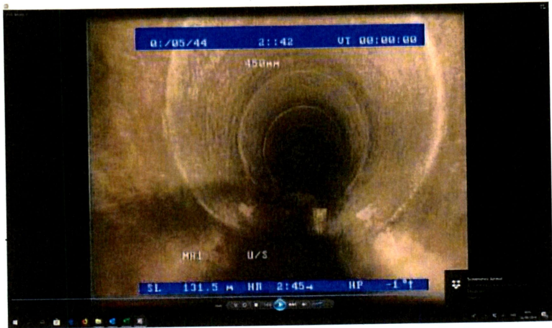
Distance 131.5m Debris in pipe. No Connections
