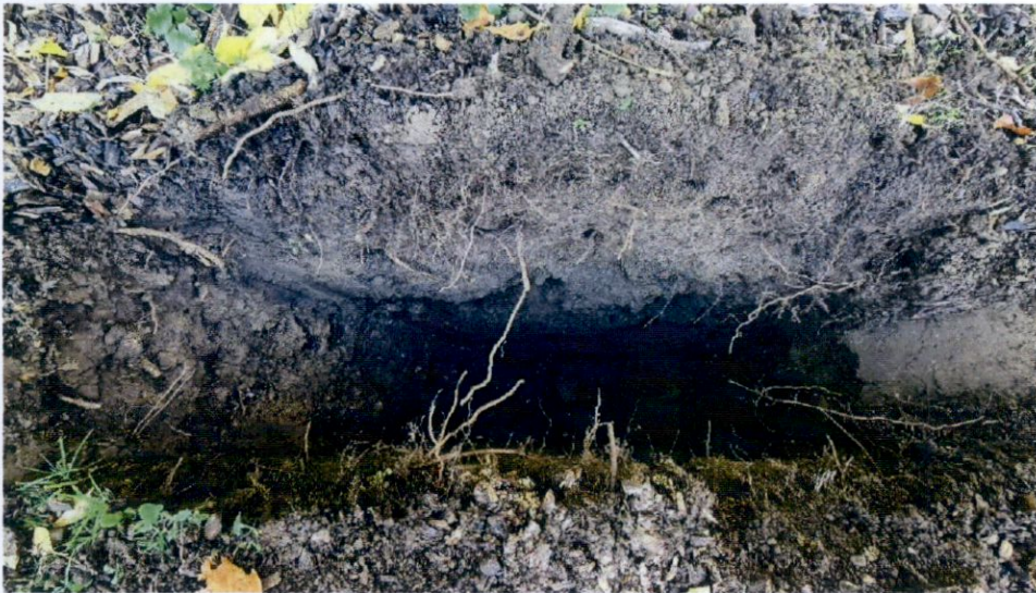
Fig 7. Infiltration test pit 24-11-2022
