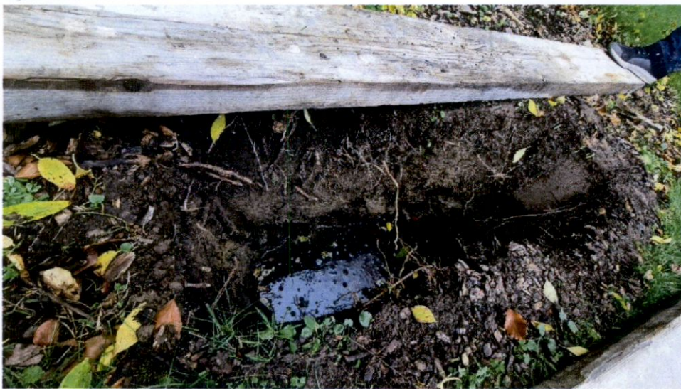
Fig 10. Infiltration test pit 25-11-2022
