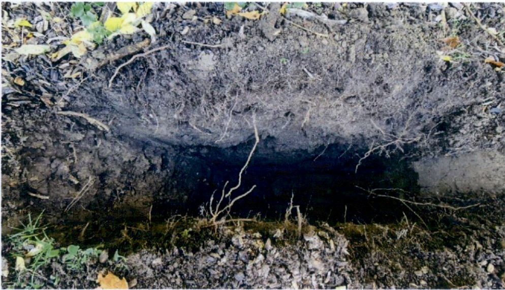
Fig 11. Trial Pit- Depth 1.2m BCL
