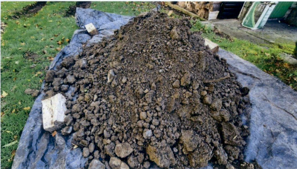
Fig 12. Trial Pit-Excavated Soil
