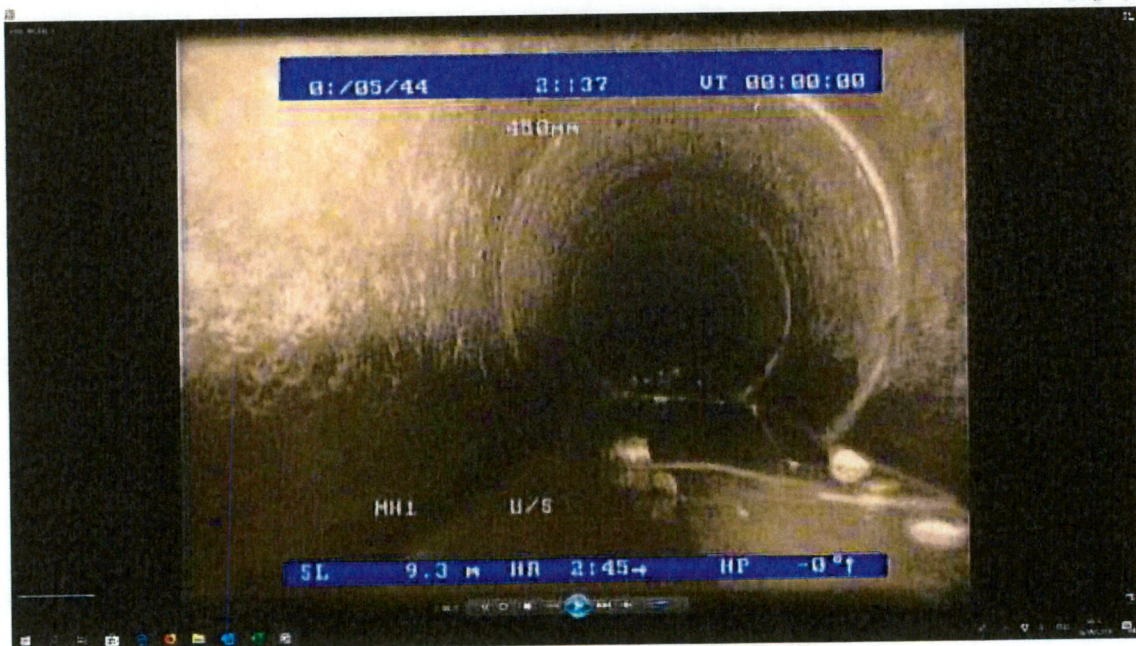
Distance 9.3m Standing water. No connections
