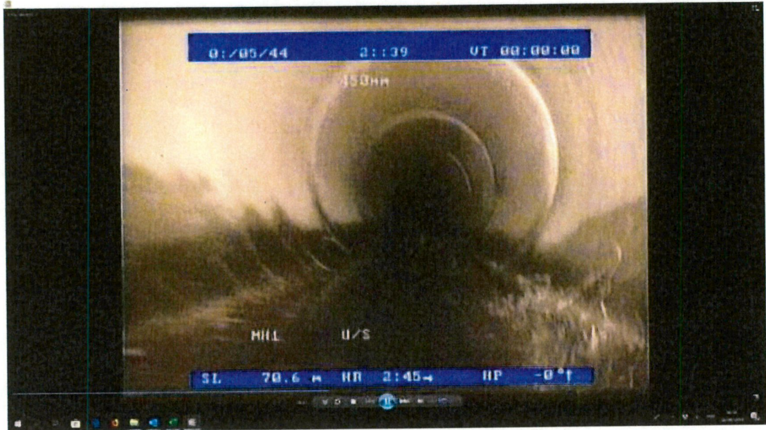
Extensive root growth. No Connections
