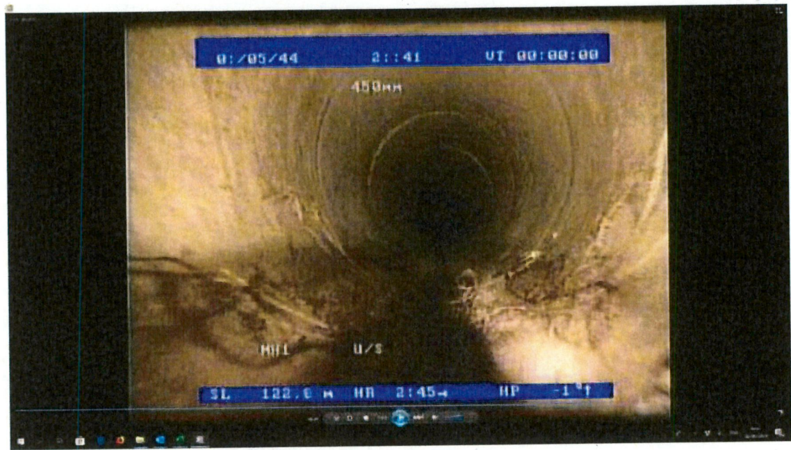
Distance 122.8m. Root growth. No Connections
