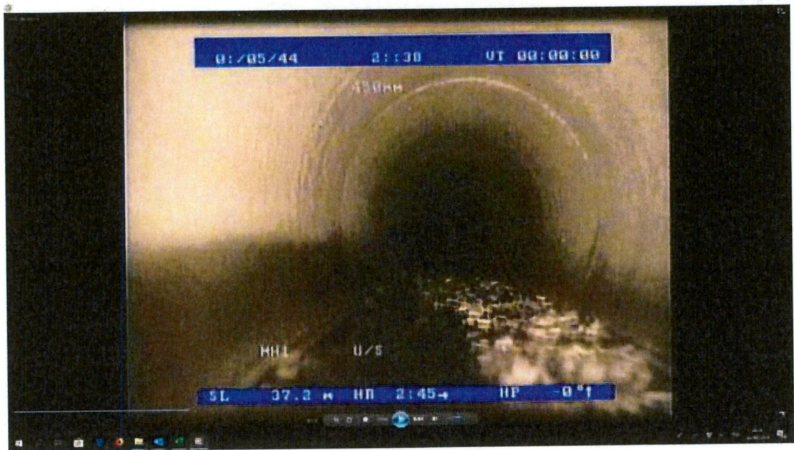
Debris in pipe. No connections
