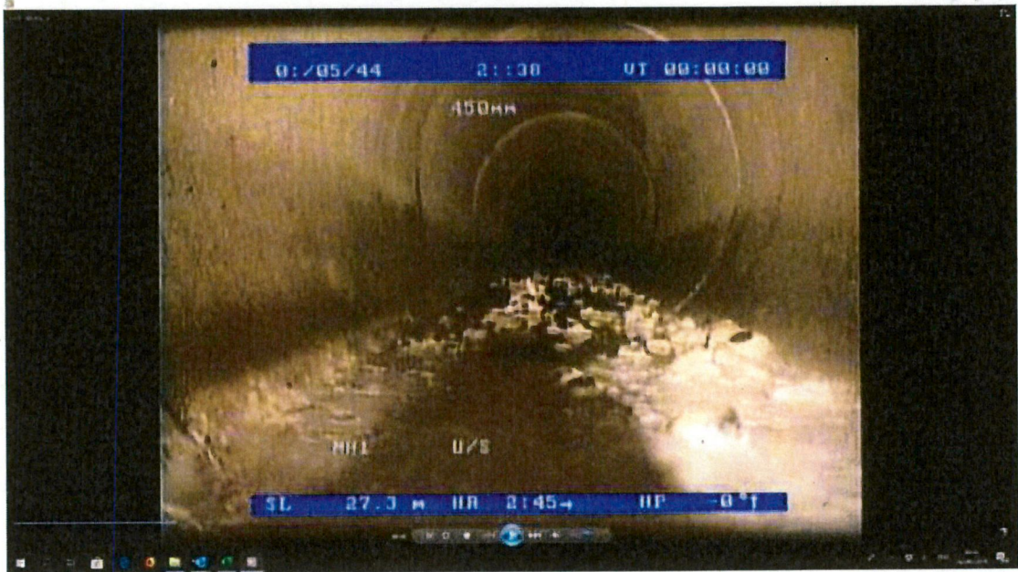
Debris & standing water. No connections
