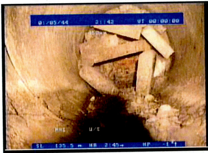
Fig. 7 - Snapshot from Camera Survey at termination.
