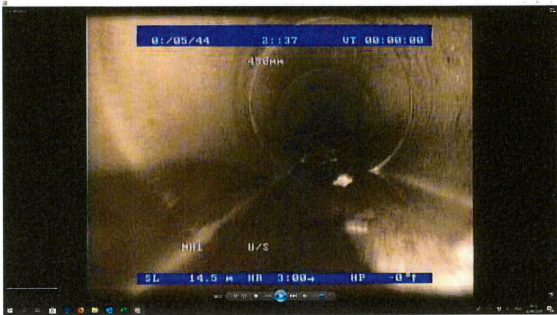
Distance 14.5m Standing water. No connections
