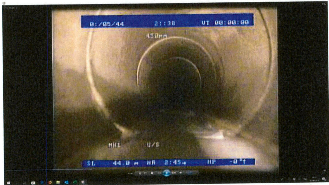
Standing water, No connections
