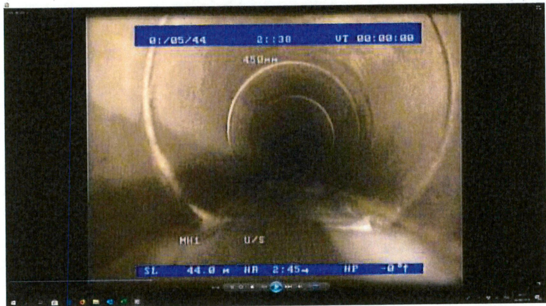
Distance 44.0m. Standing water, No connections
