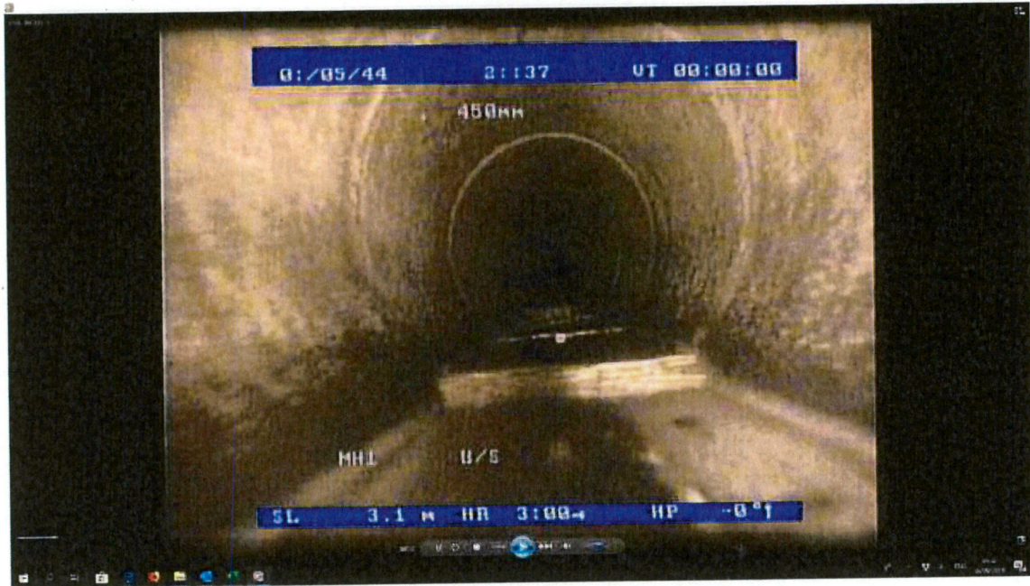
Distance 3.1m Standing water. No connection.
