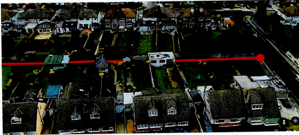
Fig 6 - Extract from google maps 3D view with the culvert line plotted, running under existing buildings
