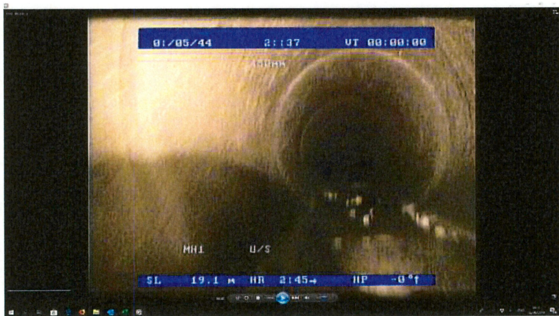
Distance 19.1m Standing water. No connections
