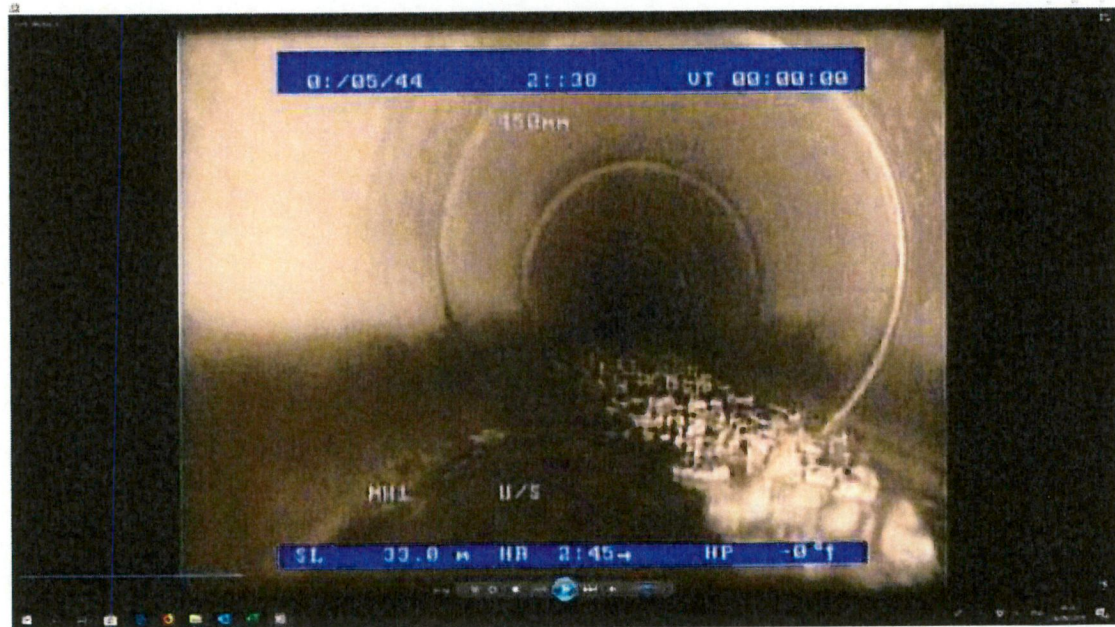
Debris in pipe. No connections
