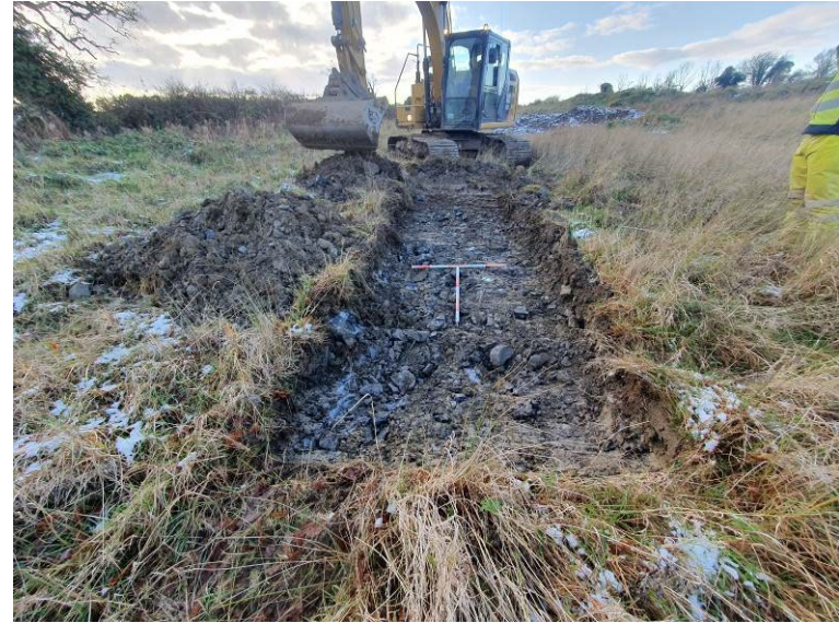
Plate 2 – Trench 2, facing southwest
