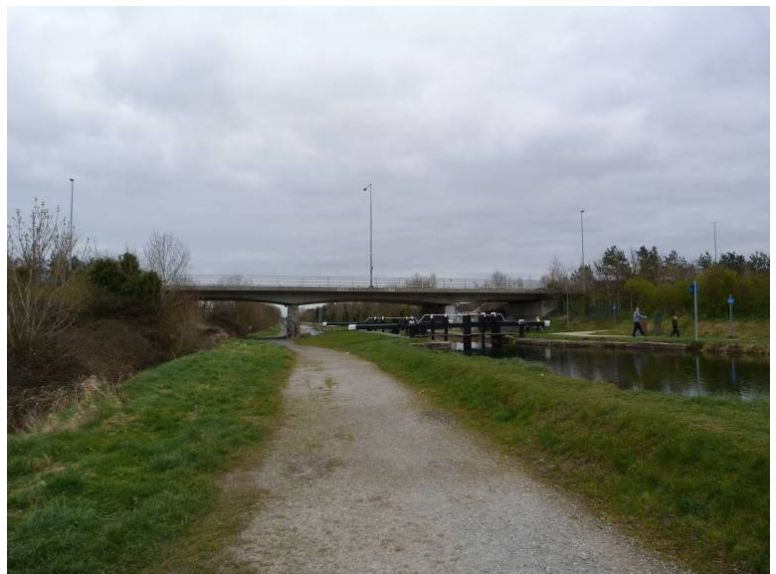
Plate 24. The Grand Canal, view to east, with bridge of R113 in background.
