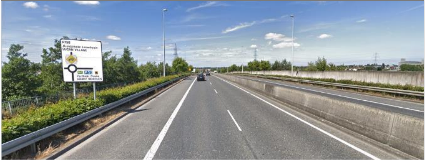
Figure 10.7 – Grange Castle Road Northbound (R136)
