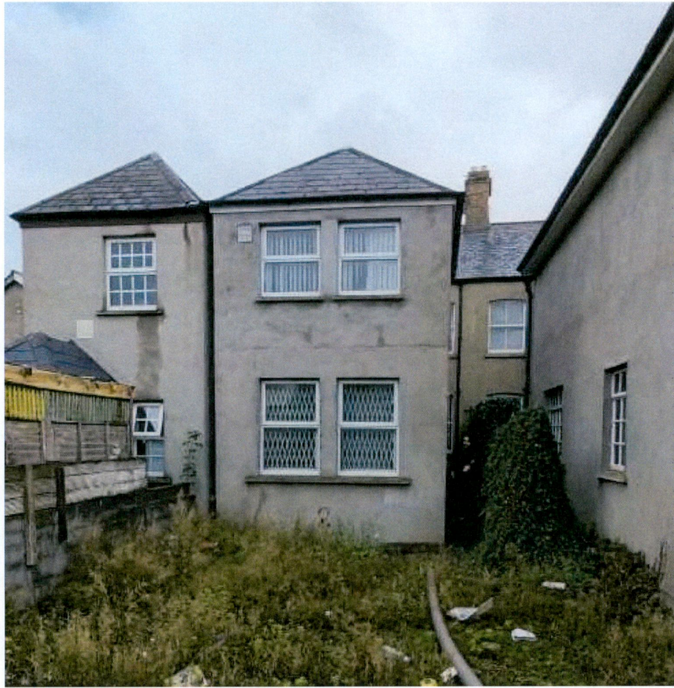
Image of rear elevation indicating the 2 storey extension built in 1997.
