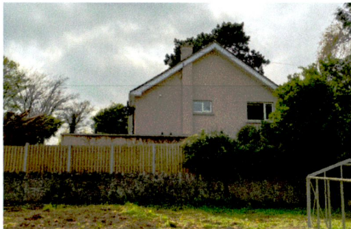
Left: view of neighbouring house to the east.
