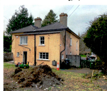
Above: East and North Elevations, April 2021 as seen from inside the NE corner of the site, this photograph was taken standing on top of a raised mound.
