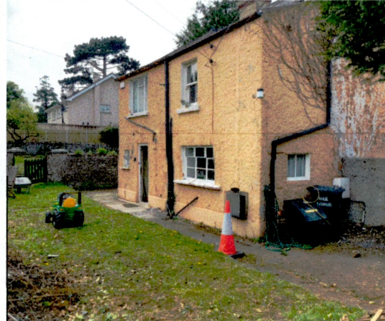
Above: North Eastern corner of the building, April 2021
